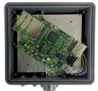
Enclosure with Mikrotik Routerboard
